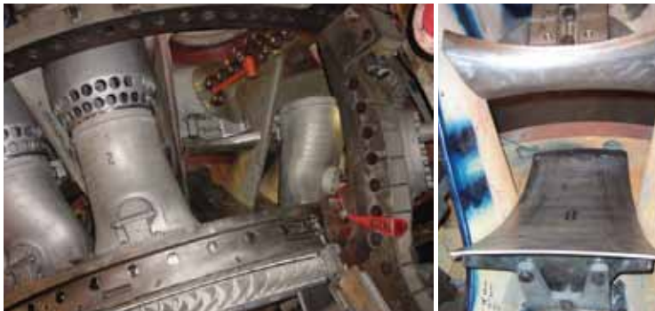
7FA-P1 Guide Vane Support Welding
