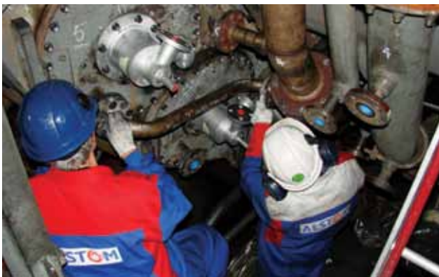
Figure 5. Inspection Work on Frame 9E Turbine
